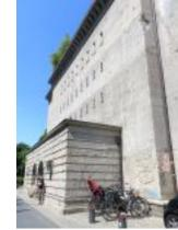
The listed air raid bunker was constructed during the second world war... The building could house up to 3000 seated people distributed on five floors during air raids... a 1,8 meter thick outer concrete wall and a 3 meter thick concrete ceiling. In the year 2003 an art collector bought the bunker and commissioned Jens Casper of Realarchitektur to design a place for him and his family to live in and house his collection.
