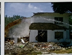
The House Demolition, 2004.
